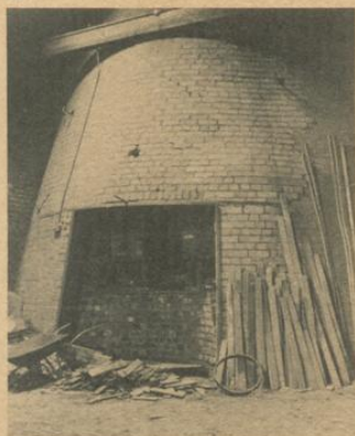
A Doncaster cementation furnace with charge material
